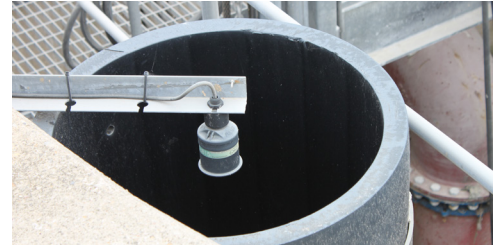
dB transducers work in conjunction with the Quantum 3 to calculate 'time to spill'
