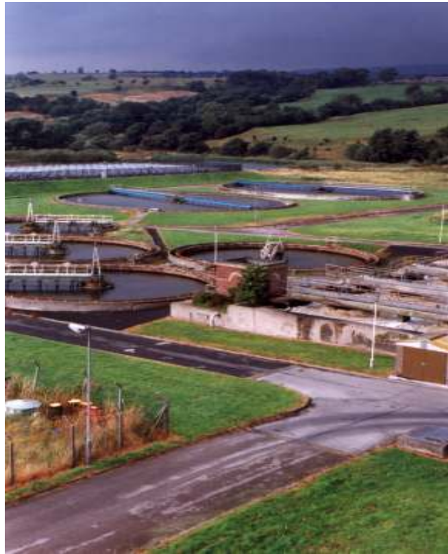
Sludge Blanket Monitoring System
